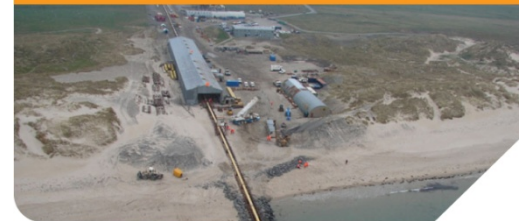
Wick Fabrication Site, UK
