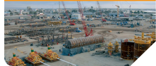
Lobito Fabrication Site, Angola
