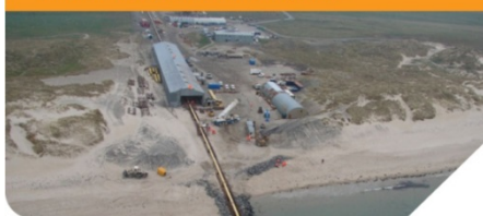
Wick Fabrication Site, UK
