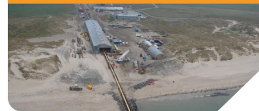
Wick Fabrication Site, UK
